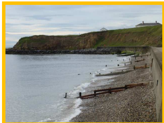
Remnants of groynes (/0102C01)
