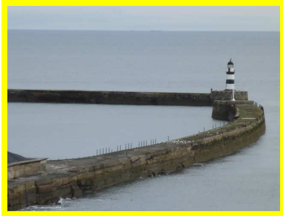
Seaham Harbour South Pier (/0104C17)
