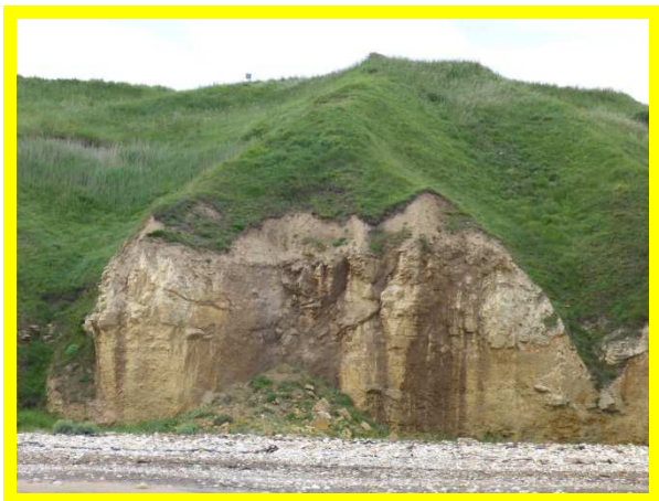
Local rock fall in cliffs (/0301C01)
