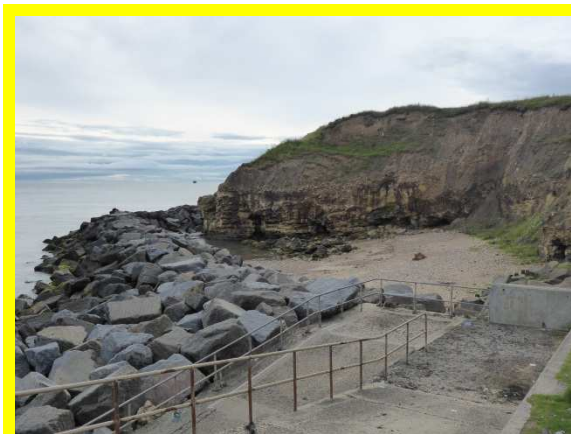
Rock berm around Featherbed Rocks headland (/0103C01)
