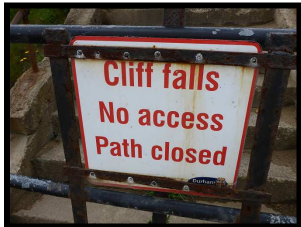
Closed access steps (/0301C01)
