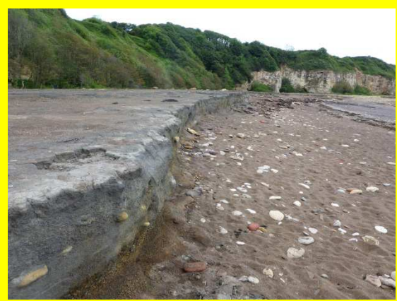
Residual spoil beach at Hawthorne Hive (/0201C01)
