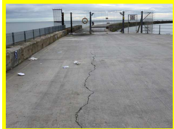
Deck of Seaham Harbour North Pier (/0104C03)
