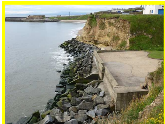
Rock berm around Dawdon Dene culvert and further south (/0103C01)
