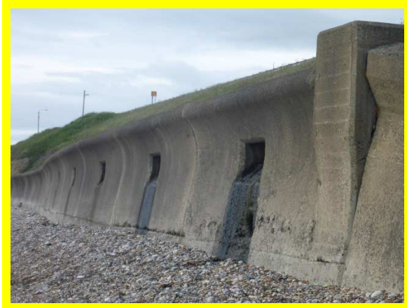
Seaham sea wall (/0102C01)
