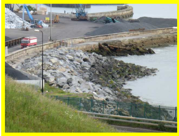
Tipped rubble (/0104C16) and rock revetment (/0104C01)
